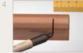
Mark the insertion depth on the tube.
