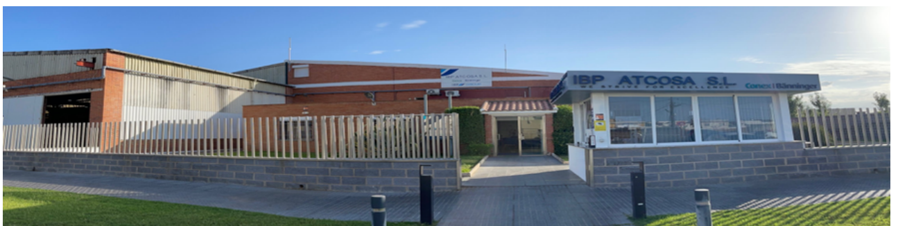
IBP ATCOSA, Poligono Industrial, Quintos-Aeropuerto production plant in Cordoba (Spain).
